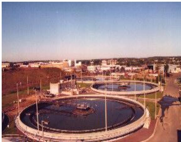
Fig-2, Secondary clarifiers in a wastewater treatment plant:-
