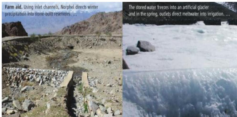
FIGURE 2. Artificial glacier introduced by C. Norphel. Source: Norphel, 2009
